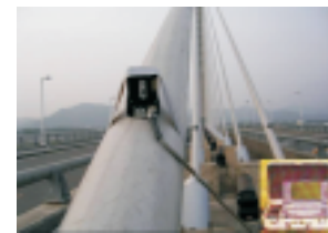
Figure 3-2 Verification of the repair of Gi-Lu Cable-stayed bridge in Nantou County after earthquake damage
