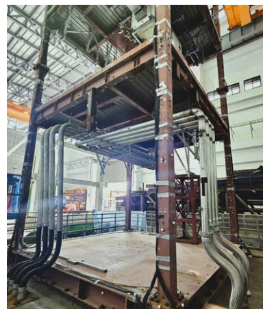
▲ Test specimen of first-floor suspended utility pipelines.
